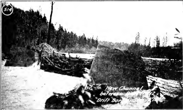
FIG. 10.—NEW CHANNEL BETWEEN PIERS NOS. 11 AND 12 OF DRIFT BARRIER.
